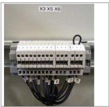
When an alarm occurs, the X3 relay contacts are de-energized and switch.
